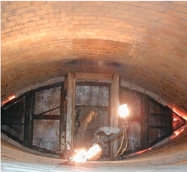
Installation of the heat shield
